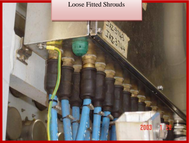
PROBLEM Tight bending radius and corrosion
